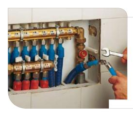
Connect the new pipe to the damaged one with the R576 traction fitting.
