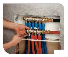
Once the pipe is cut with the right lenght, proceed with the connection to the manifold. Ends of the pipe are protected with the covers R998.
