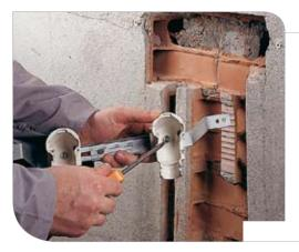
After selecting the required position on the wall for drains and pipes, proceed with the assembly of the fittings using the correct brackets.
