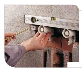
Correct position of the connections is done using a sprit level.
