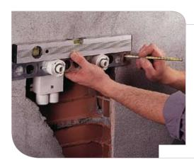
The bar is set to the wall using expansion dowels and a spirit level for the correct position.
