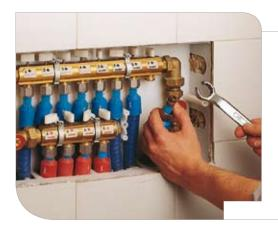
Close the lockshield, untighten the nut of the adaptator and disconnect the pipe to be replaced.
