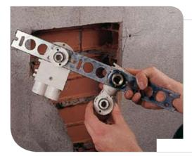
Position the fittings to the bar with the desired interaxis.
