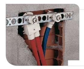
When the assembly is carried out, perform a pressure test, and after that block the fittings and the protection covering of the sleeves with concrete.
