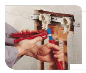
For a correct positioning of the fittings, it is necessary the pipe is cut precisely and perpendicularly with cutters R990.
