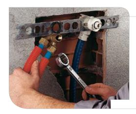
Once the bar is fixed, proceed in connecting the pipes to the fittings.
