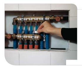
When assembly is carried out, set the single circuits with R73K key.
